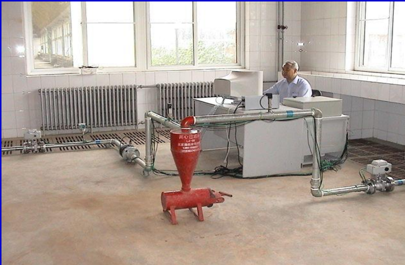
Automatic tester for flowrate-pressure
